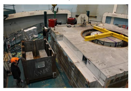
Figure 5: Lifting of one of the cut blocks to a DD type 2 steel container
