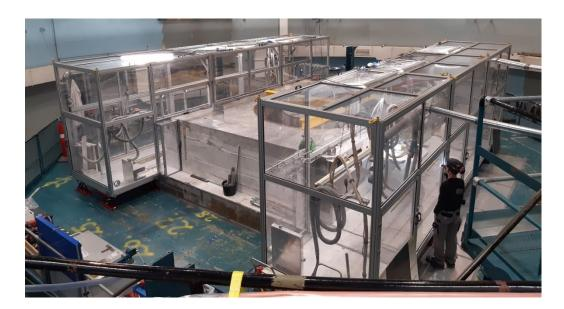
Figure 4: Dust containments mounted on facade 1 and 3. Ventilation ducts for the dust containments are connected to the vacuum extractors at the ground level.
