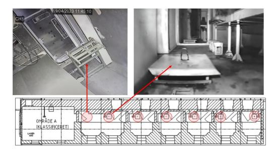
Figure 21: Steel rack and ventilation filter covers in the hot cells
