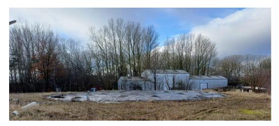
Figure 31: One of the basins with cover with heavy-duty tarpaulin material
