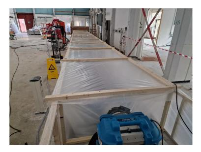
Figure 28: The custom-made enclosure placed over the opening in the deck over the crawl space and the connected environmental box with HEPA-filters.
