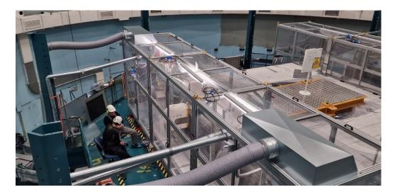
Figure 7: The new recirculation of the ventilated air in the dust compartments.
