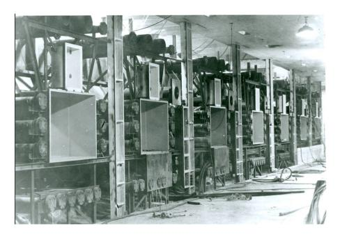
Figure 11: Picture form the construction of the Hot Cell Facility in the 1960's showing some of the now embedded cables and tubes.
