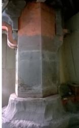
Figure 9: Shot concrete on the back side of the ISB.
