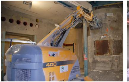
Figure 8: Removal of shot concrete from the ISB next to the  $D_2O$  plant room by use of a scabbler on a Brokk.
