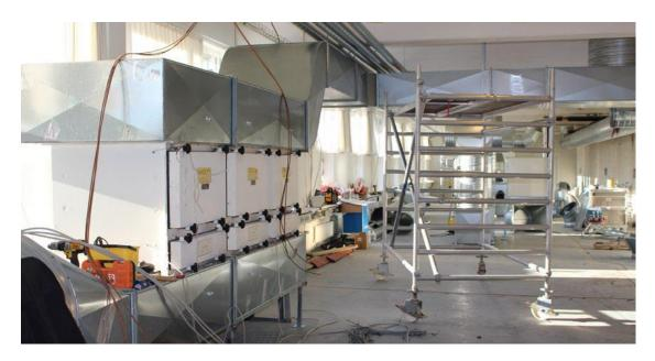
Figure 21 : Filters from the roof are now placed inside the facility
