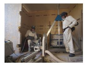
Figure 30: Wall shaver during shaving the ceiling in the powder room
